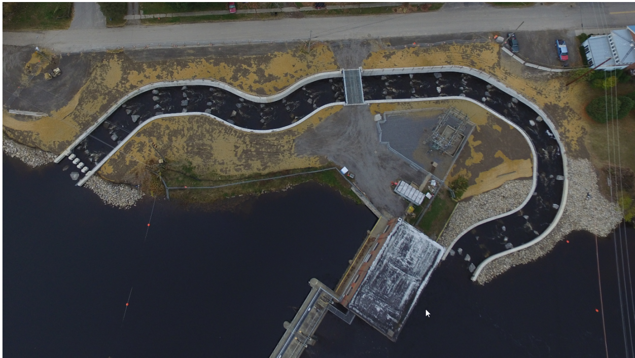
Figure 3. Nature-like fishway on the Oswegatchie River in New York.
