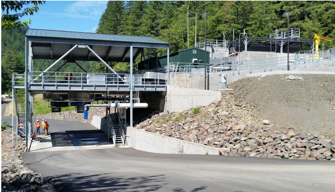
Figure 12. Overview of Adult Collection and Sorting Facility at North Fork Dam
