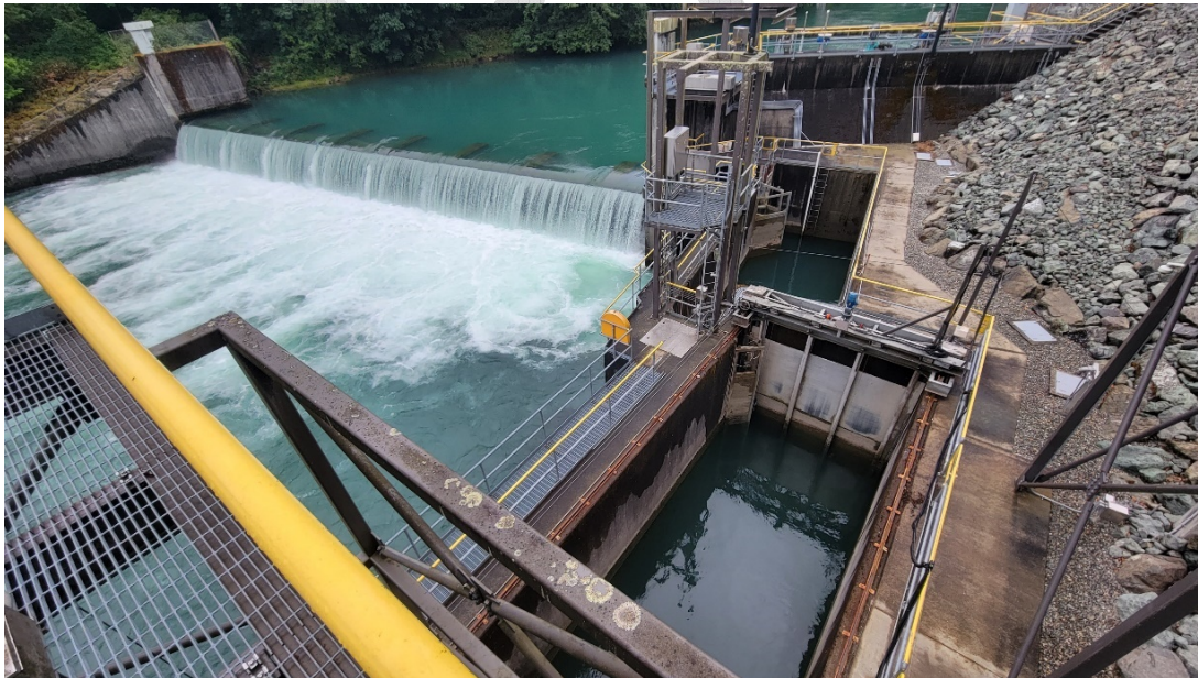
Figure 11. Lower Baker River Adult Trap and Transport Facility: Barrier Dam and Collection/Crowding Gallery
