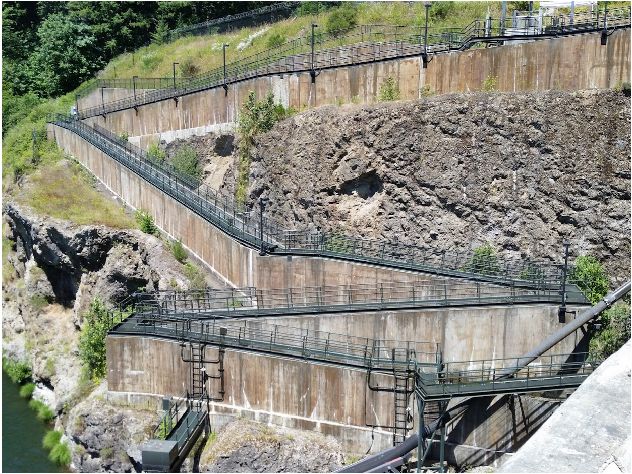
Figure 5. River Mill Dam Half Ice-Harbor Baffle (pool, weir, and orifice) Fish Ladder
