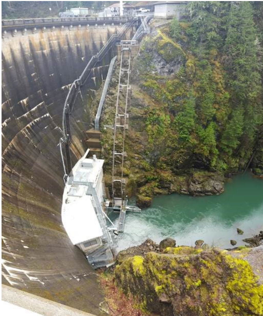
Figure 7. Skokomish Dam No. 2 Adult Collection Facility Fish Lift
