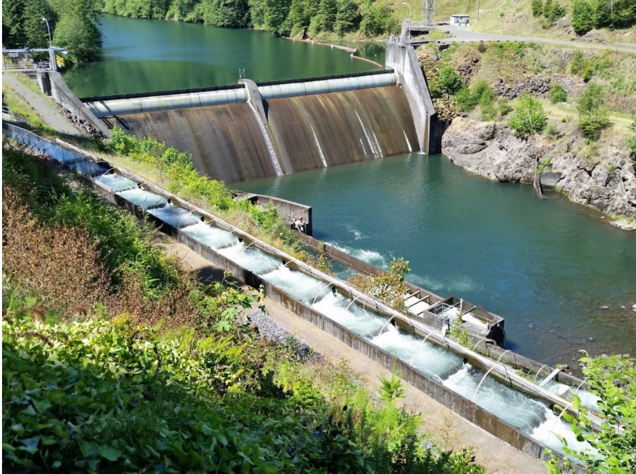
Figure 4. Faraday Diversion and North Fork Dams' 2.1-Mile-Long, Half Ice-Harbor Baffle (pool, weir, and orifice) Fish Ladder
