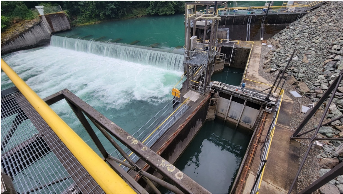
Figure 11. Lower Baker River Adult Trap and Transport Facility: Barrier Dam and Collection/Crowding Gallery
