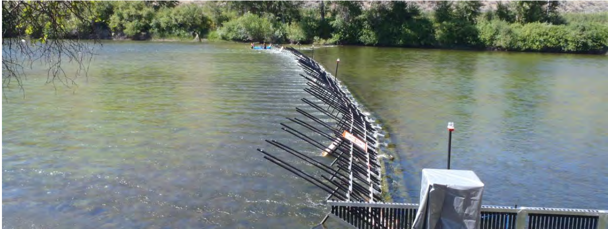
Figure 16. Picket Barrier on the Okanogan River Operated by the Chief Joseph Hatchery
