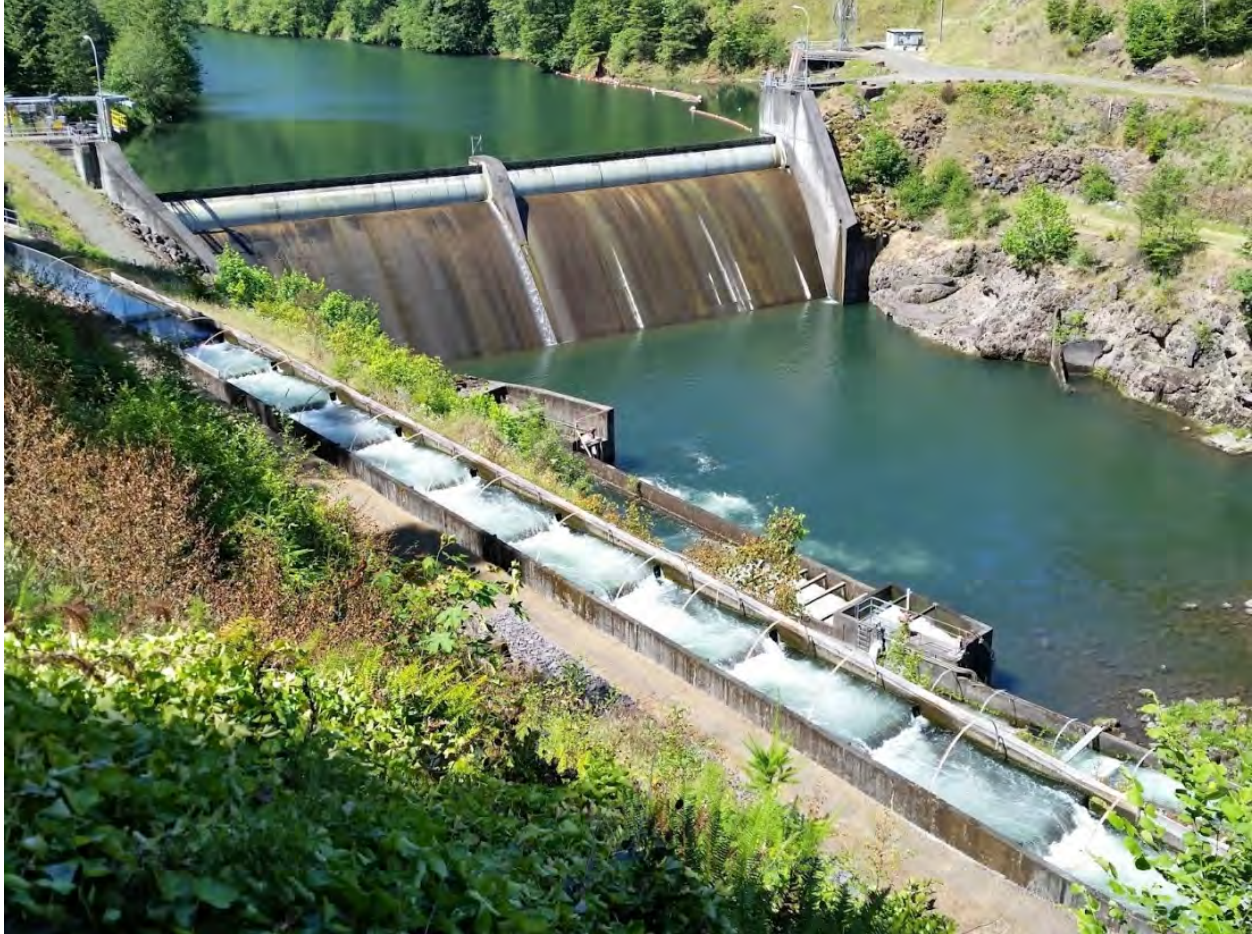
Figure 4. Faraday Diversion and North Fork Dams' 2.1-Mile-Long, Half Ice-Harbor Baffle (pool, weir, and orifice) Fish Ladder
